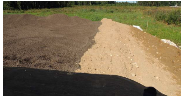
h) Construction of LWA layer at sec 4. (25.8.2015)
