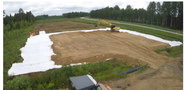
b) Construction of embankment sec. 1 (20.7.2015)
