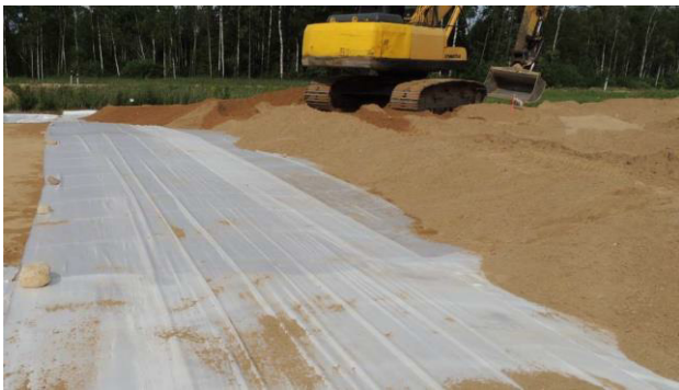
c) Installed upper reinforcement, sec. 2 (21.7.2015)
