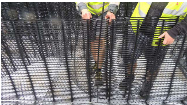
e) Construction of Geocell structure at sec. 3. (31.7.2015)
