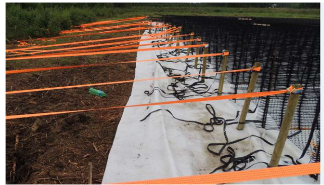
d) Construction of Geocell structure (31.7.2015)
