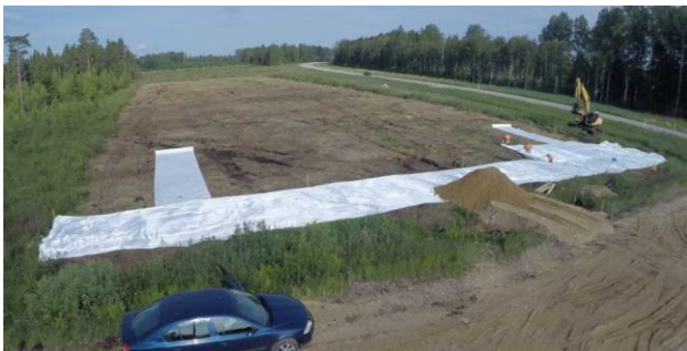
a) Start of construction of sec. 1 (20.7.2015)
