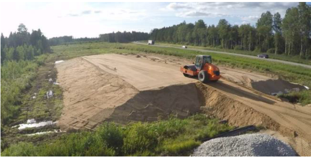
g) Compaction of the embankment. sec.1 (24.8.2015)
