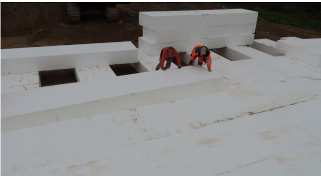
i) Installation of EPS-blocks at sec. 5 (16.9.2015)
